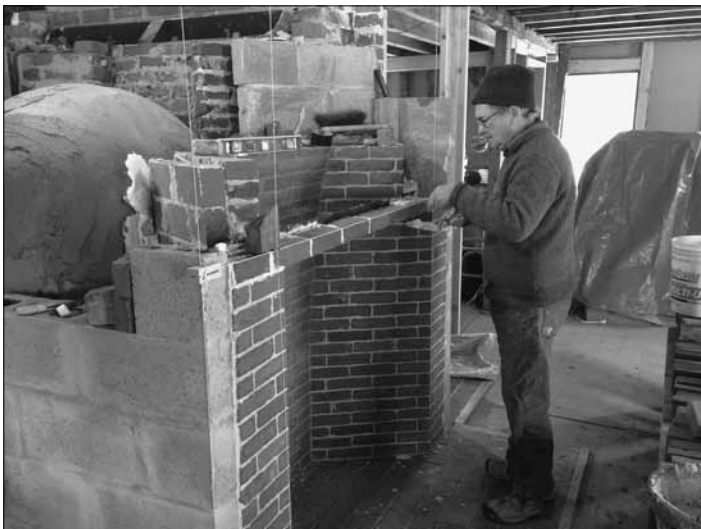
Left: Peter Moore working on the west fireplace. The dome on the left side of the photo is the exterior of the bake oven. Right: The completed east fireplace with the bake oven and crane.
